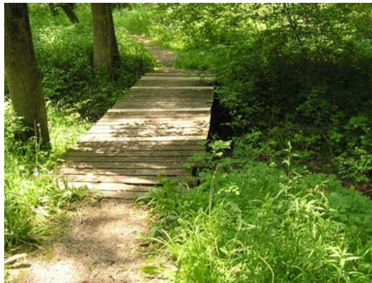
Bridge 3, footbridge at overflow
