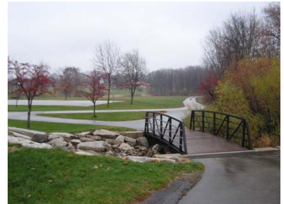
Bridge 4, metal span
