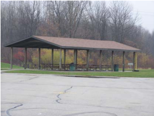
Meadowbrook Park Open Air Shelter
